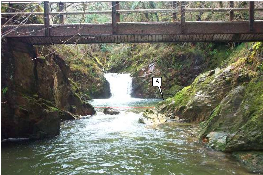
Figure 7: Afon Wen hydrograph recording site. The water depth recorder is located in the pool at location A. Flow is measured at the pool outlet along the section shown in red.
